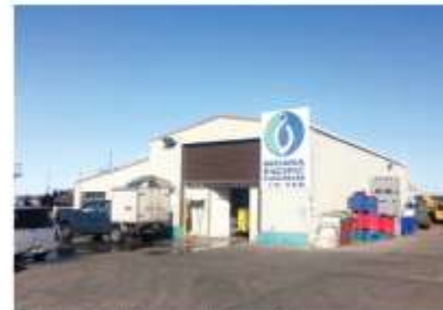
Existing Building (north facade)
