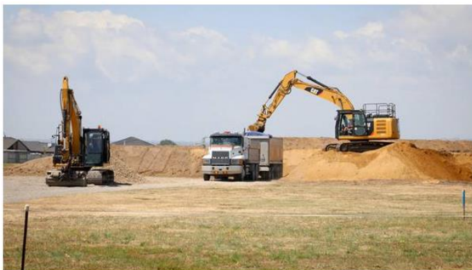
Diggers remove the stockpiled fill in Golden Sands in December. Photo / Andrew Warner
